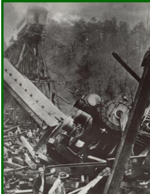
Trestle collapse at Panther Creek in 1898.
