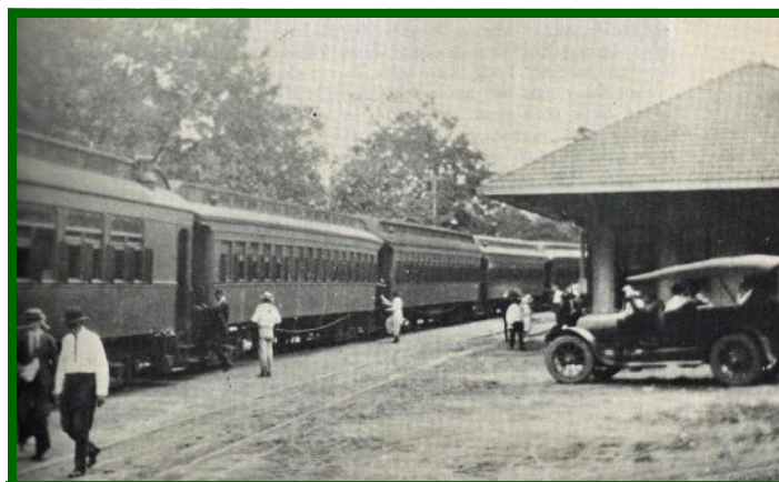
A Moss family photo of the Tallulah Falls Railroad depot in the 1920s.
